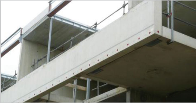
FIXING OF BALCONY RAILINGS
